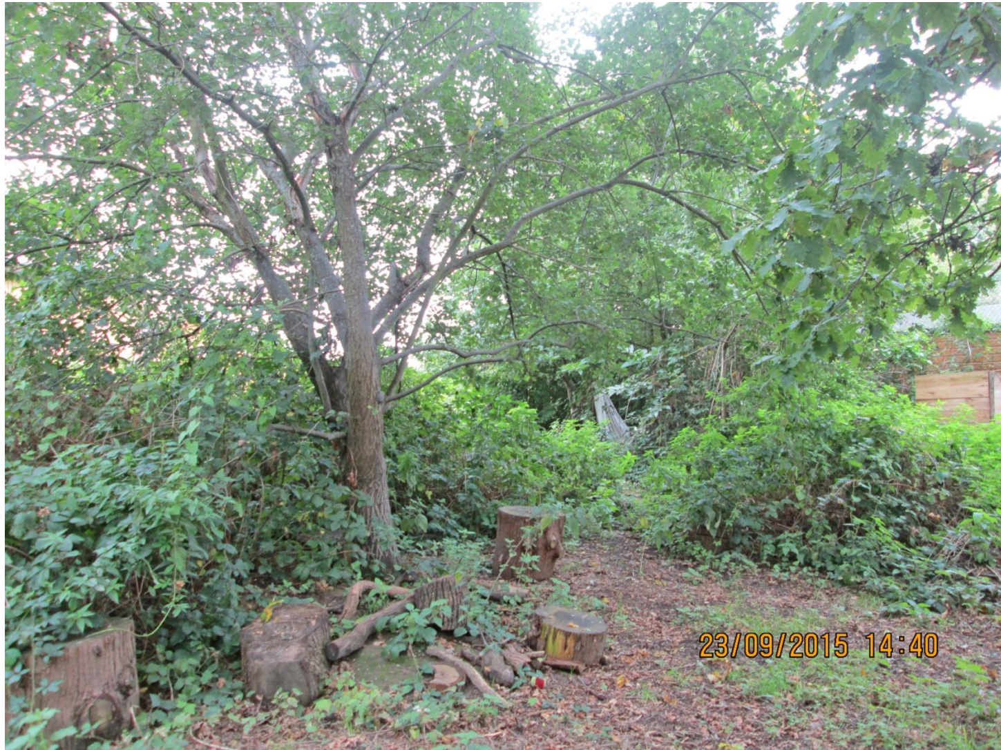
Figure 4 : Wooded area at west end, part of construction access route and compound
